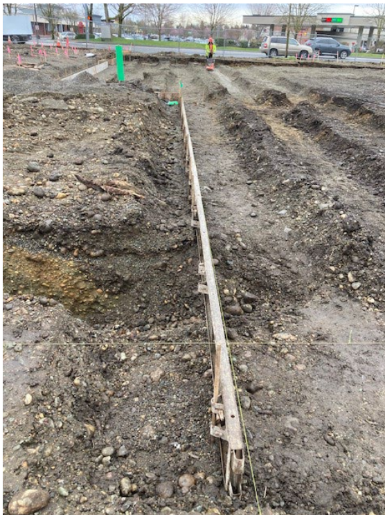
Figure 1: Progress of footings and foundation wall installation at Lakewood, WA
