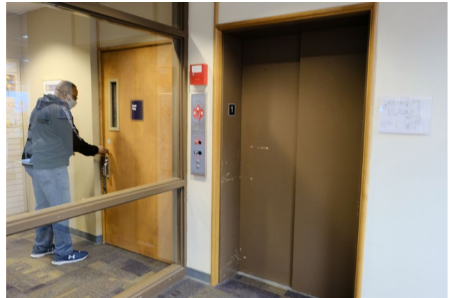
Entry Lobby and Elevator
