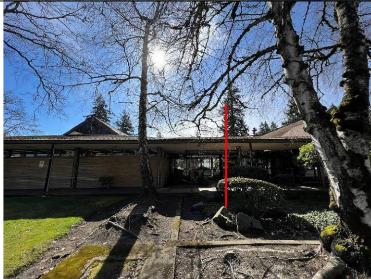
Photograph 71: Area to the left of the red line appears to be the 1974 addition.
