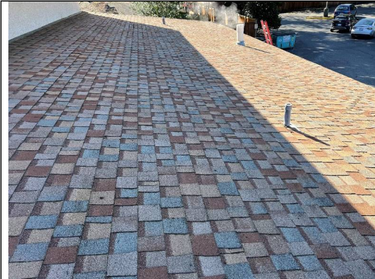
Photograph 22: Looking laterally across the Tamko architectural laminate shingles.
