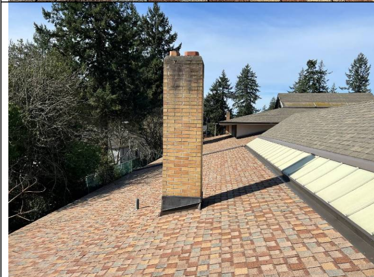
Photograph 57: Chimney penetration flashed with sheet metal flashing.
