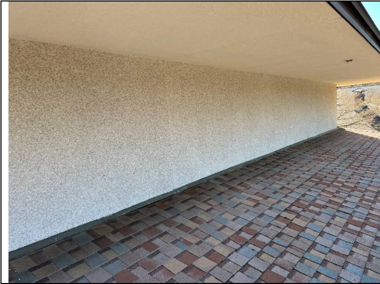
Photograph 31: Typical marblecrete clad rising wall above the lower roof.
