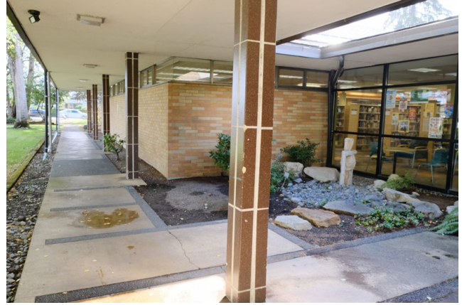
Courtyard near entry
