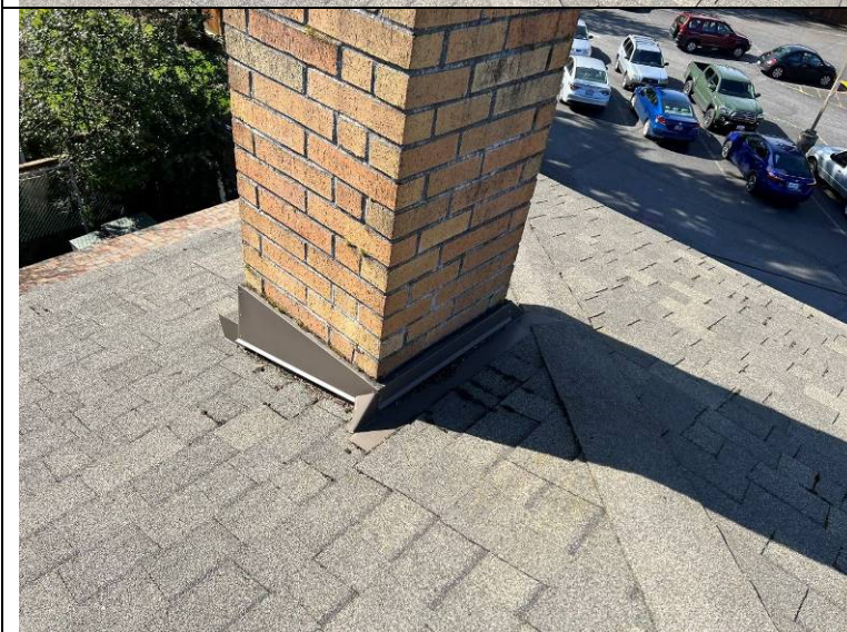
Photograph 93: Closer view of the sheet metal chimney flashing.
