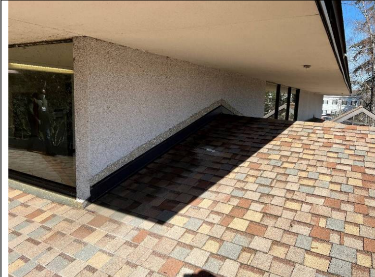
Photograph 32: Roof to wall transition along a rake wall.
