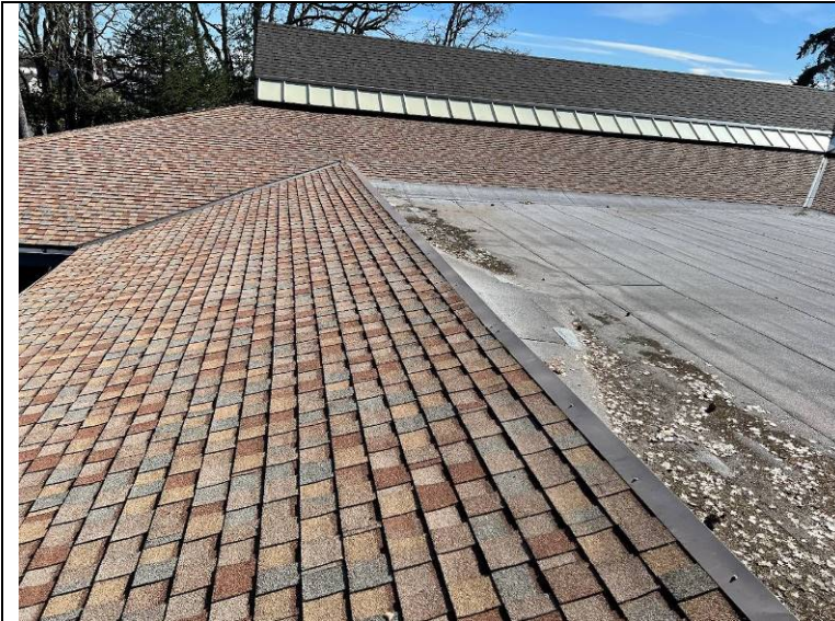
Photograph 43: Steep slope to low slope roof transition.
