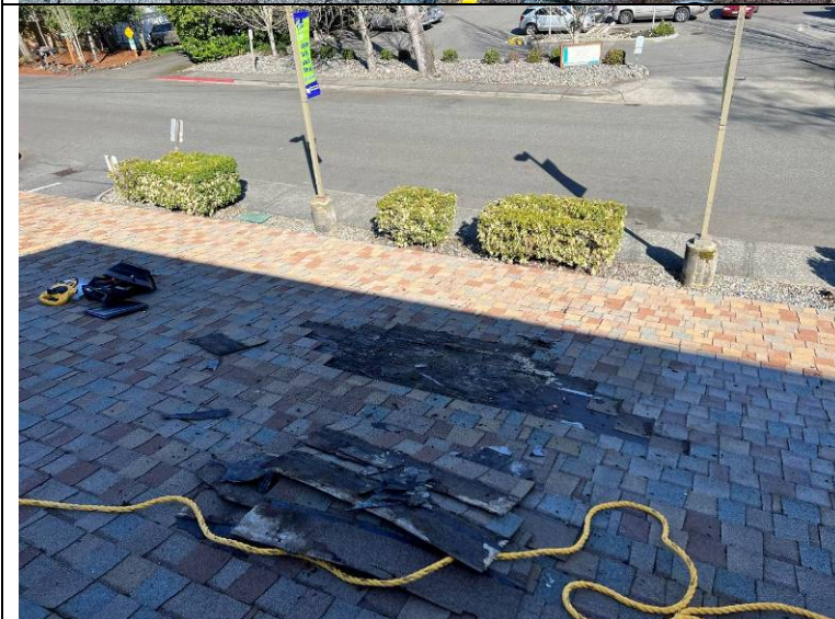
Photograph 9: Overview of test opening location #2.
