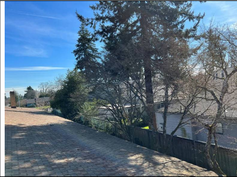
Photograph 40: Overview of the south sloping roof and trees within close proximity of the roof.
