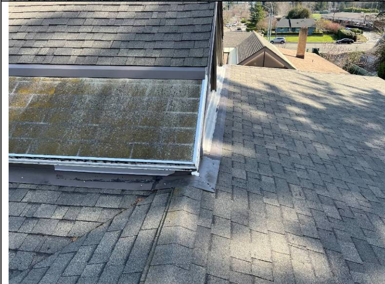
Photograph 86: Roof to skylight transition.
