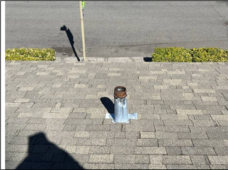
Photograph 97: Pipe penetration flashed with a lead flashing.
