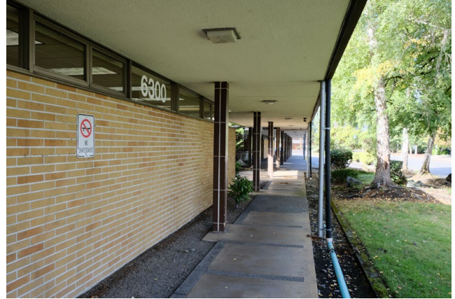
Roof overhang at north side
