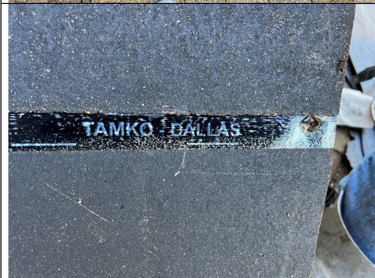
Photograph 24: Tamko label on the backside of one of the removed shingles.
