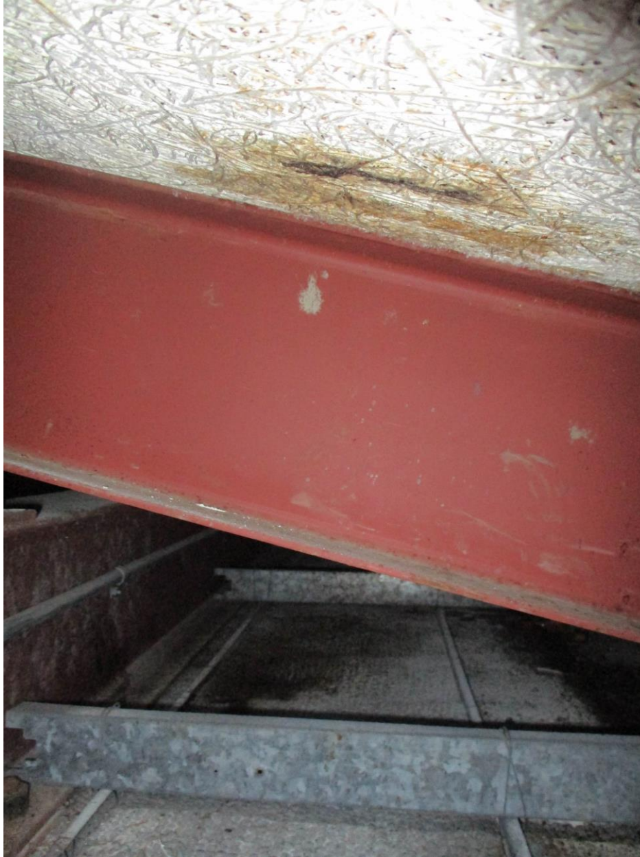
Photo 4 - Structural Steel Beams & Soffit Framing
