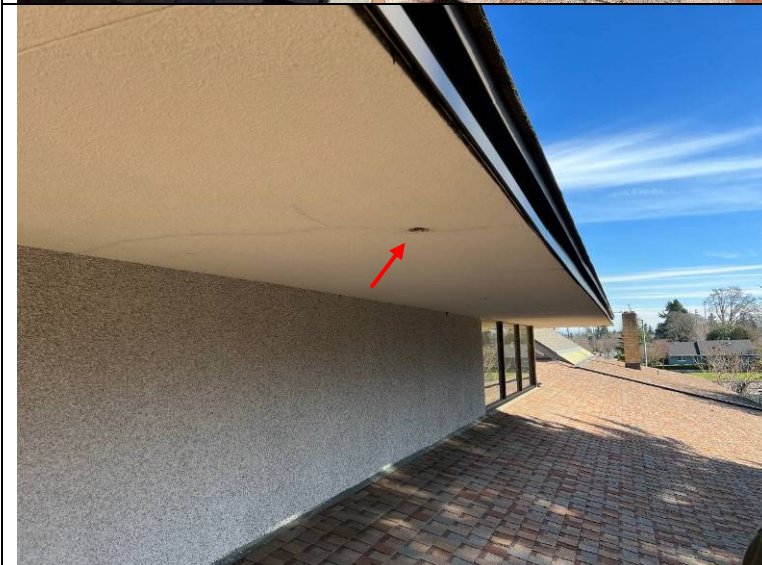
Photograph 102: Soffit above the low roof.
