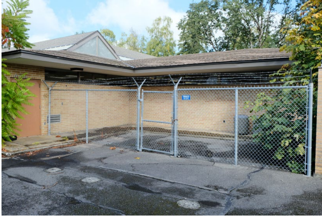
Fenced area at NE presents a security problem
