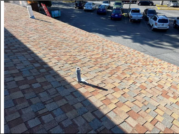
Photograph 34: Typical pipe penetration flashed with a lead penetration flashing.
