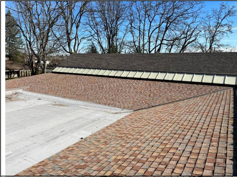
Photograph 82: Steep slope to low slope roof transition.
