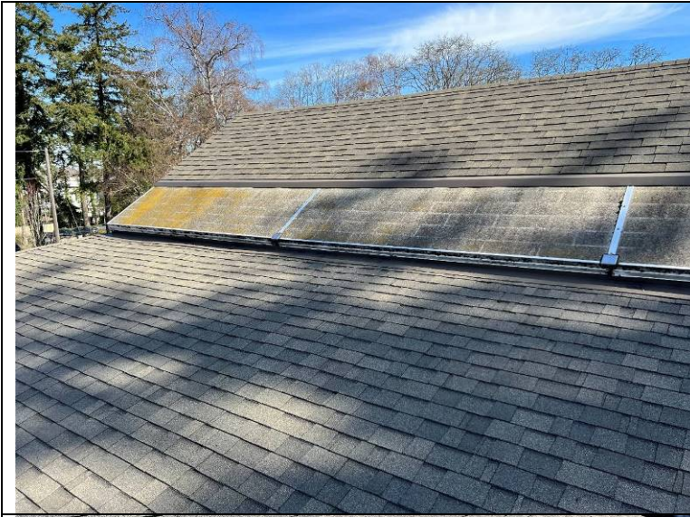
Photograph 88: Overview of the skylights at the upper roof.
