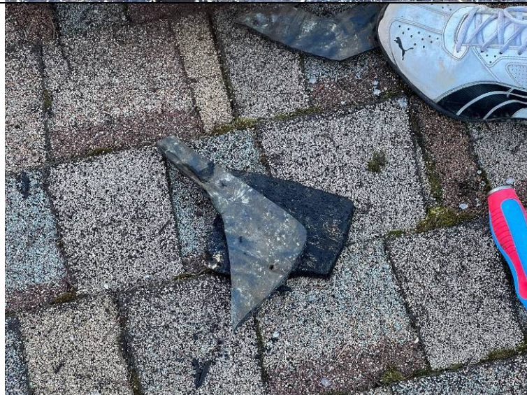
Photograph 15: Asphaltic membrane with a polyethylene surfacing.
