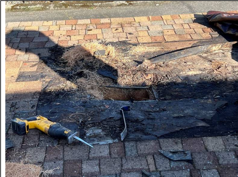
Photograph 16: Alternate view of test opening #3.
