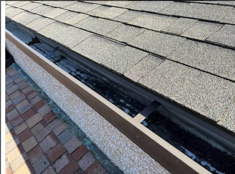
Photograph 99: Closer view of the gutter and draining edge shown in Photograph 98.
