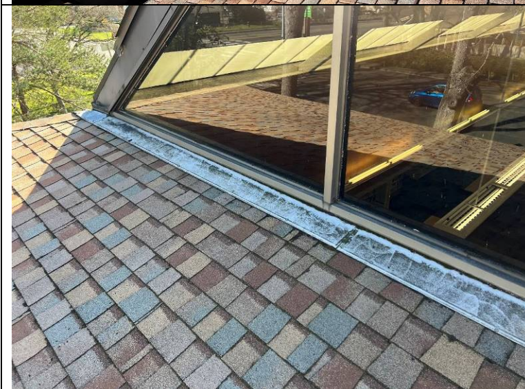
Photograph 45: Roof to clerestory transition.
