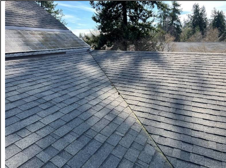
Photograph 85: Typical closed cut valley at the upper roof.
