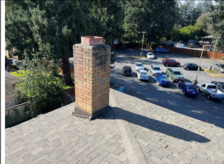
Photograph 92: Chimney penetration at the upper roof.
