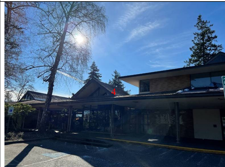
Photograph 3: Overview of the area where test opening 4 was made by Wayne's Roofing personnel.
