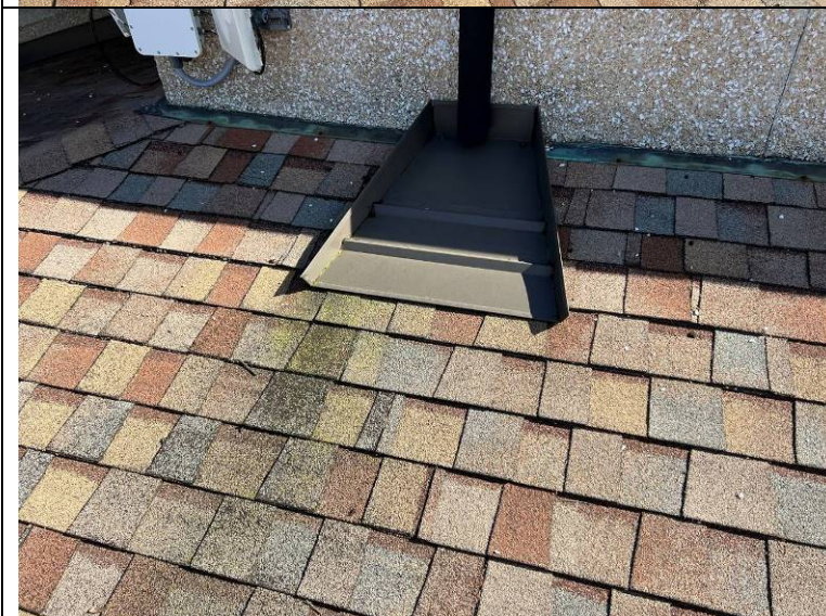
Photograph 66: Splash pad beneath the downspout from the upper roof.
