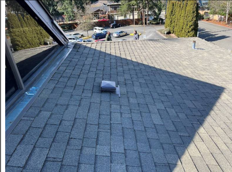
Photograph 95: Typical roof vent stripped into the shingle roof.
