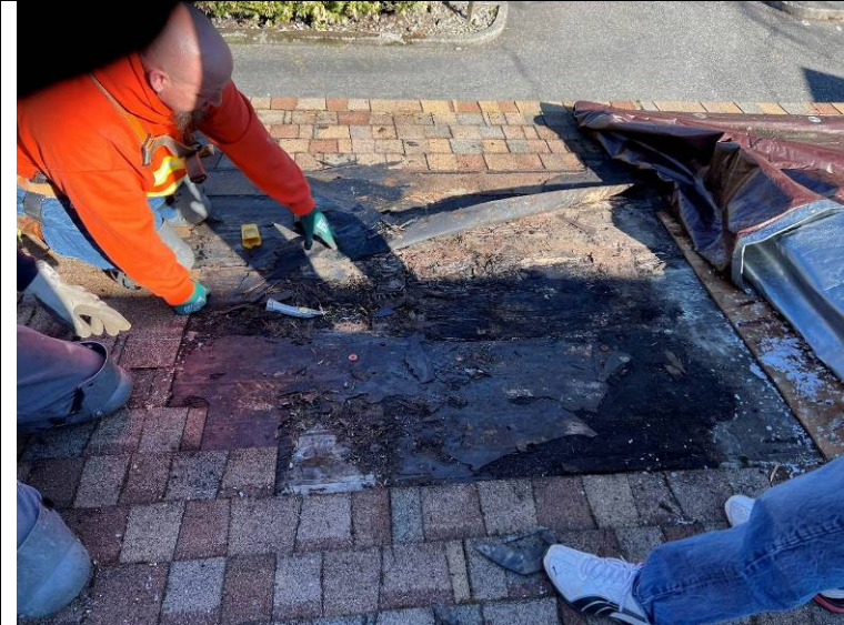
Photograph 11: Overview of opening location #3.
