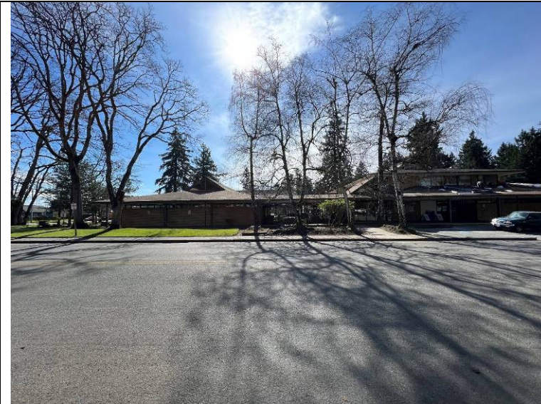
Photograph 70: Overview of the east end of the north elevation.
