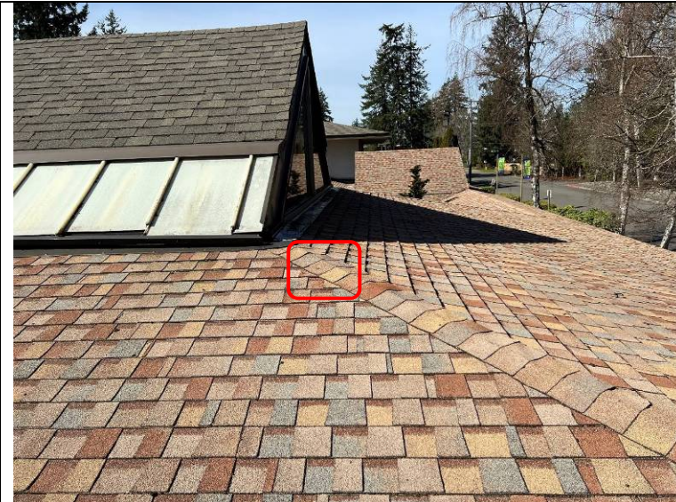
Photograph 46: Hip condition, roofed with hip shingles.
