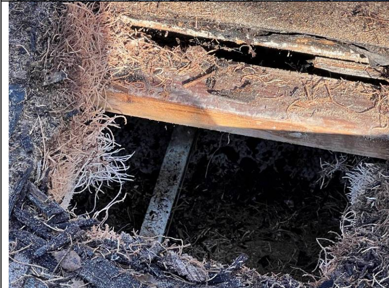
Photograph 20: Alternate view of the area shown in Photograph 19.
