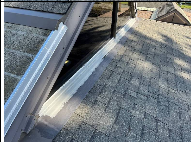
Photograph 87: Roof to clerestory transition.
