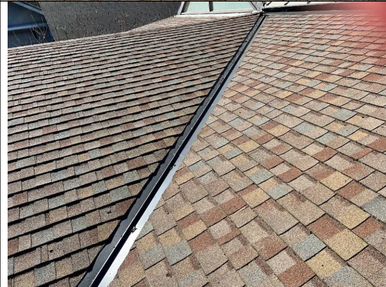
Photograph 50: Closer view of the sheet metal valley flashing.
