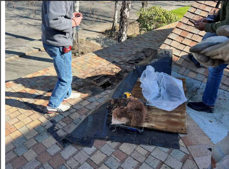
Photograph 17: Overview of test opening #4.
