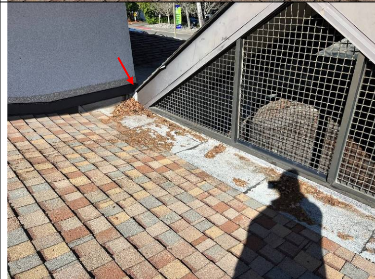
Photograph 42: Dead valley with mineral surfaced capsheet in the valley.
