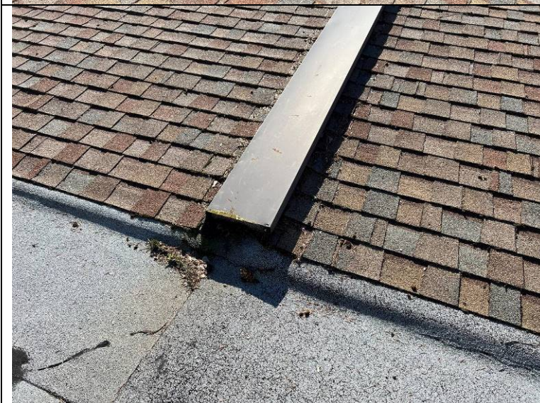
Photograph 39: Closer view of the sheet metal cover shown in Photograph 38.
