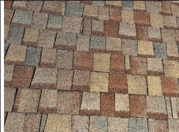
Photograph 23: Closer view of the Tamko architectural laminate shingles.
