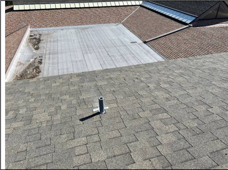
Photograph 94: Typical pipe penetration flashed with a lead.
