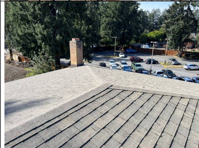
Photograph 84: Overview of the upper roof.
