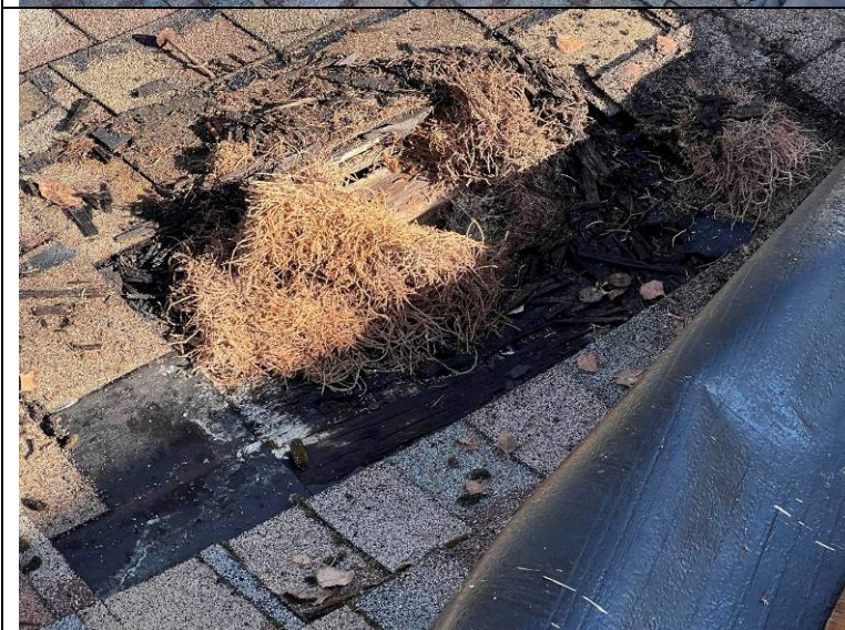
Photograph 18: Cementitious wood fiber substrate board removed at test opening #4.
