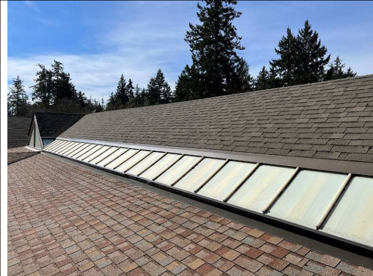
Photograph 41: Low roof to high roof transition at the translucent skylight panels.
