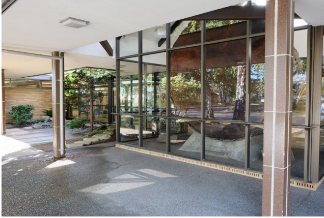
Windows near entry
