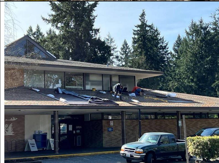
Photograph 72: Overview of the repairs at the test openings.
