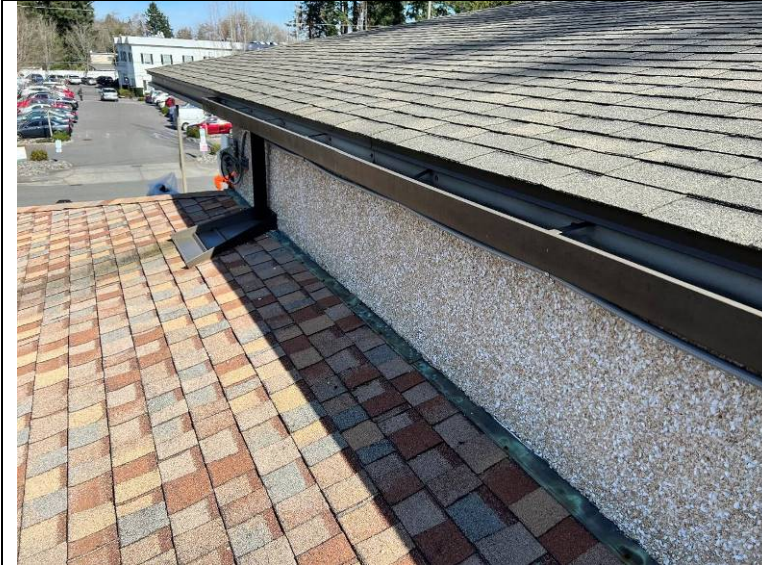
Photograph 98: Draining edge and gutter at the upper roof.
