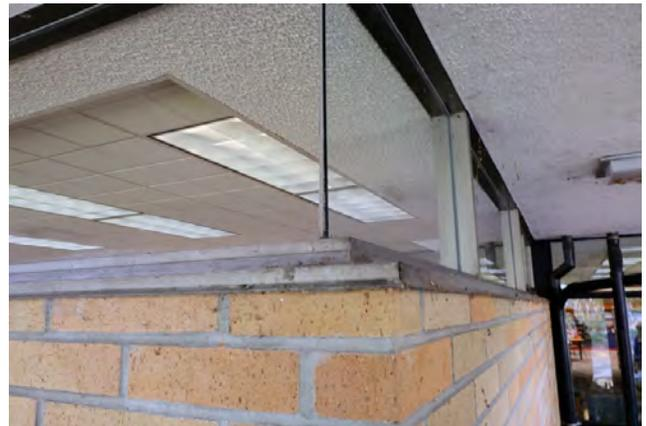
Single pane windows with failed seal at corner joint
