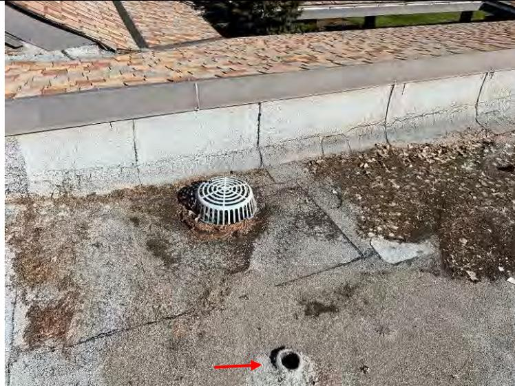
Photograph 75: Closer view of a cast iron roof drain and contractor style overflow (arrow).
