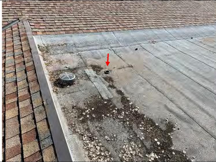
Photograph 74: Typical cast iron roof drain and adjacent contractor style overflow (arrow).
