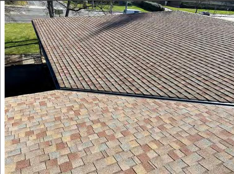
Photograph 49: Typical valley at the lower roofs configured with a sheet metal valley flashing.
