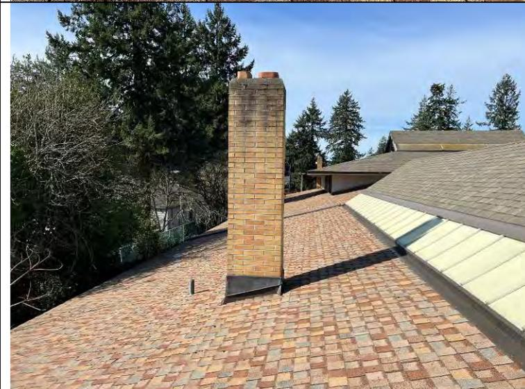
Photograph 57: Chimney penetration flashed with sheet metal flashing.
