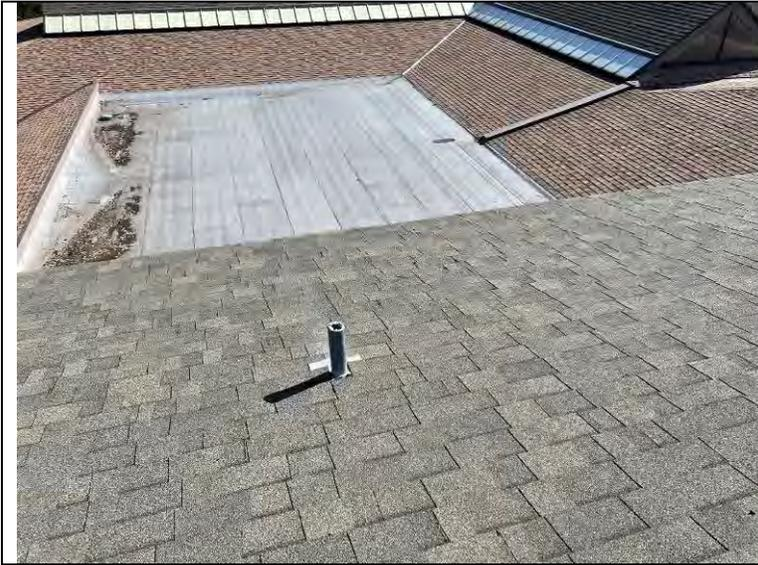
Photograph 94: Typical pipe penetration flashed with a lead.
