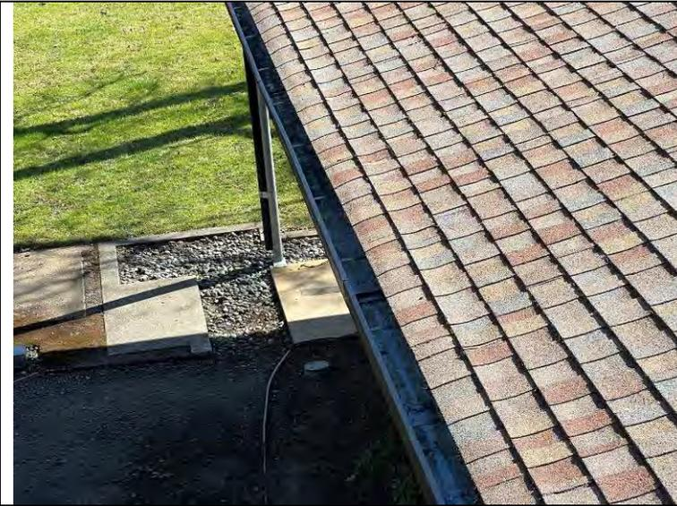
Photograph 55: Typical drainage detail with external hung gutter.
