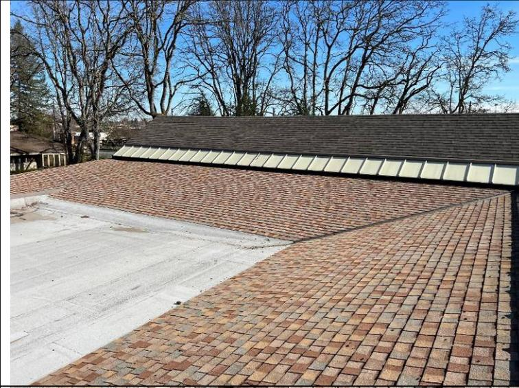
Photograph 82: Steep slope to low slope roof transition.
