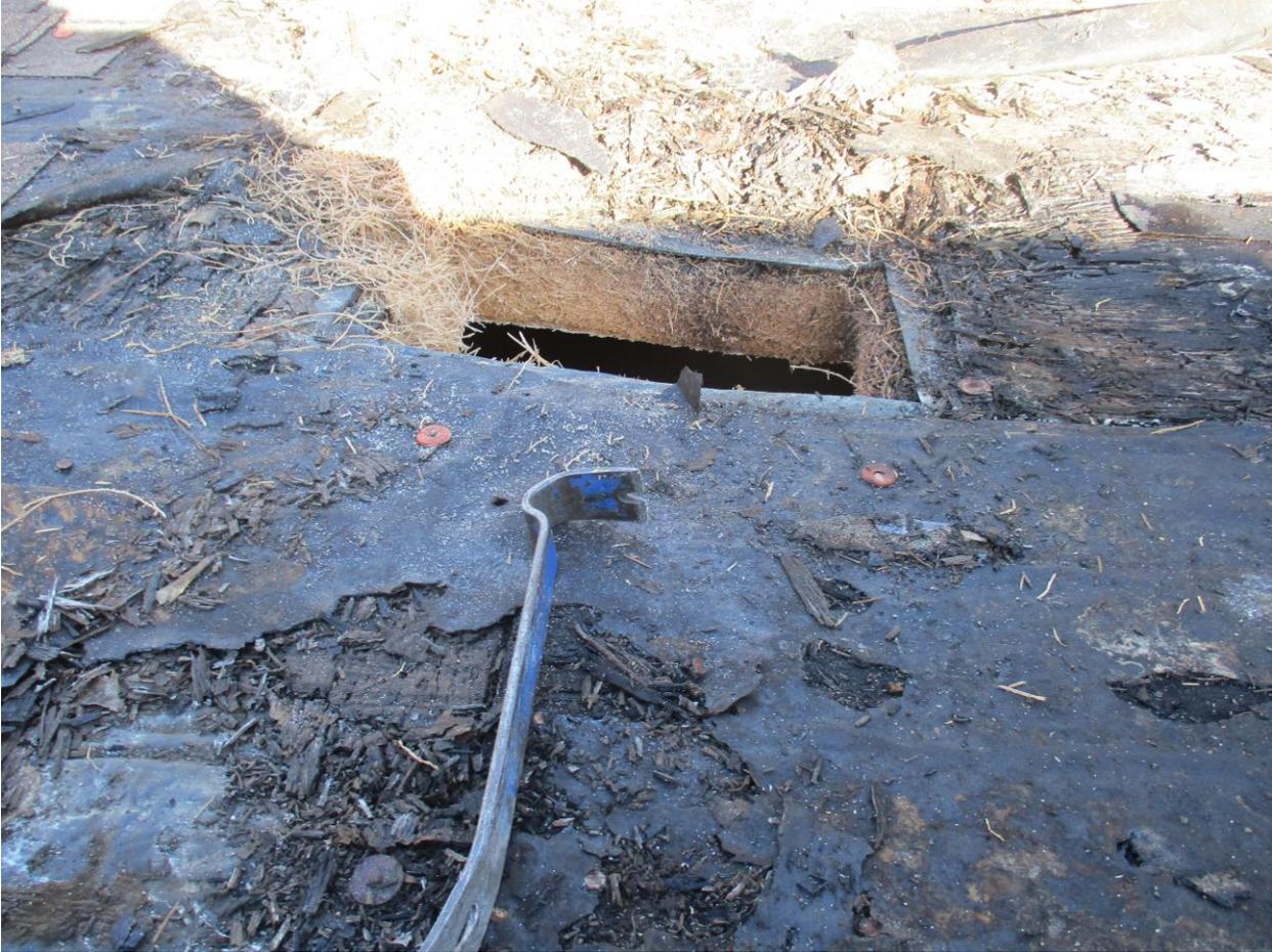
Photo 2 – Tectum Structural Panel Section
