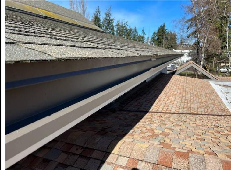
Photograph 101: Eave edge without a gutter.
