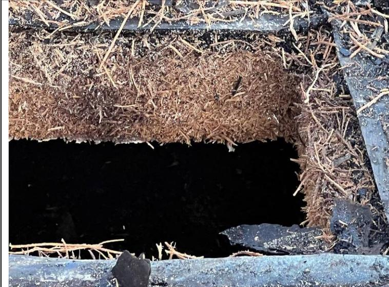
Photograph 14: Closer view of the cementitious wood fiber substrate board at the test opening.
