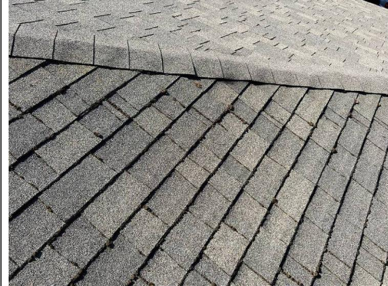
Photograph 89: Moss growth along the perimeter of the shingles.
