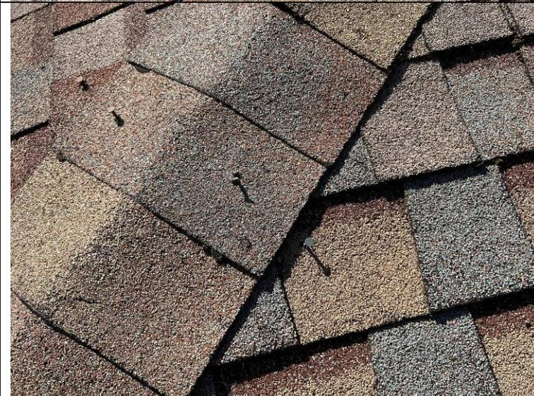
Photograph 48: Closer-up view of the backed-out nails.
