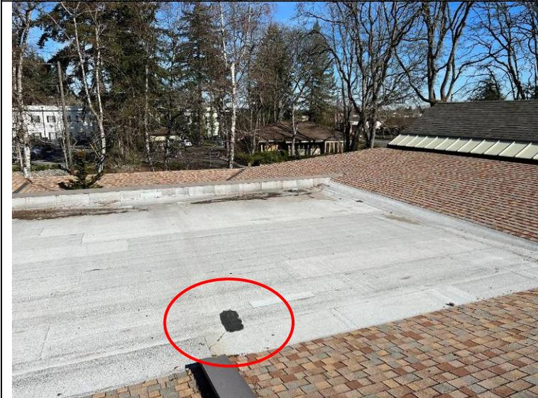
Photograph 77: Roof cement patch over an apparent location of damage.
