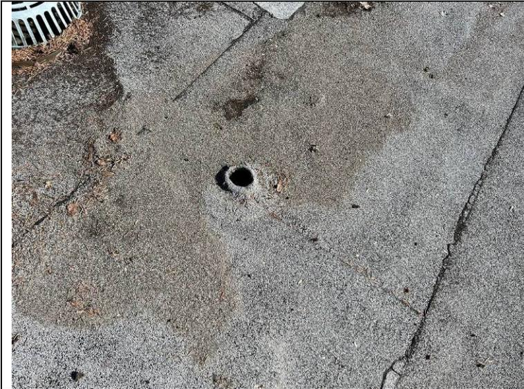
Photograph 76: Closer view of the contractor style overflow.
