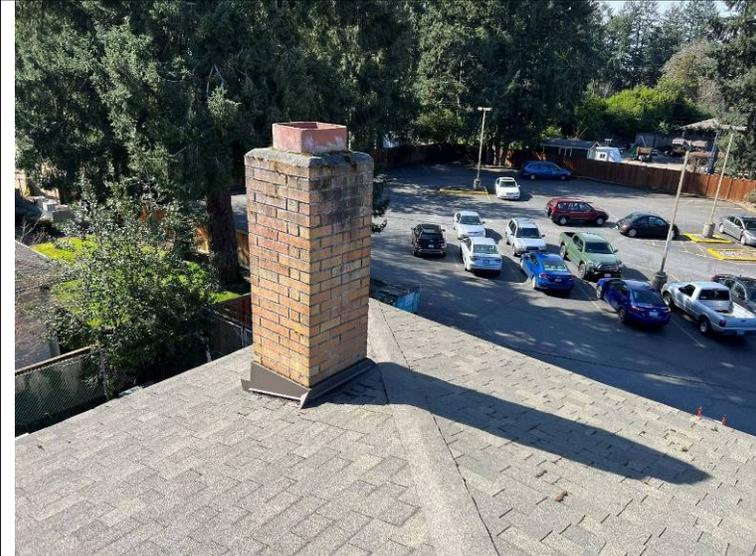
Photograph 92: Chimney penetration at the upper roof.
