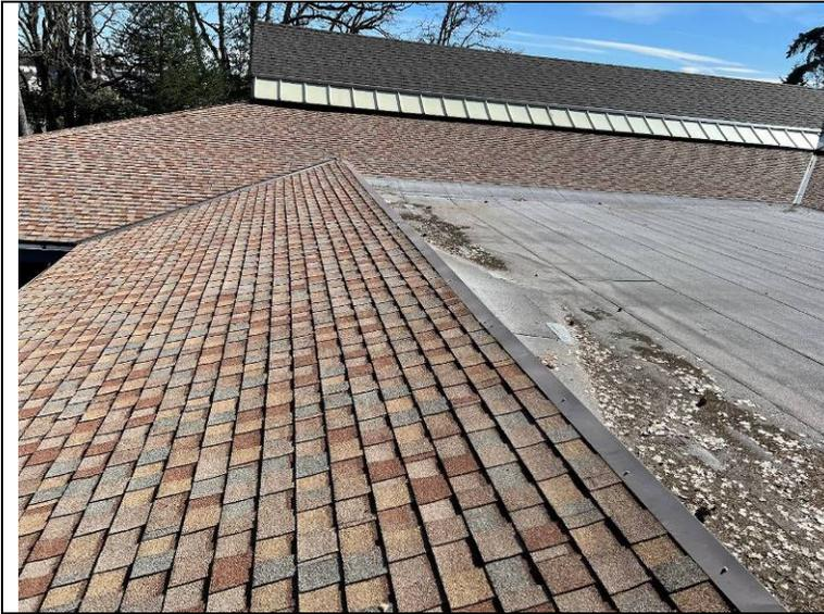
Photograph 43: Steep slope to low slope roof transition.
