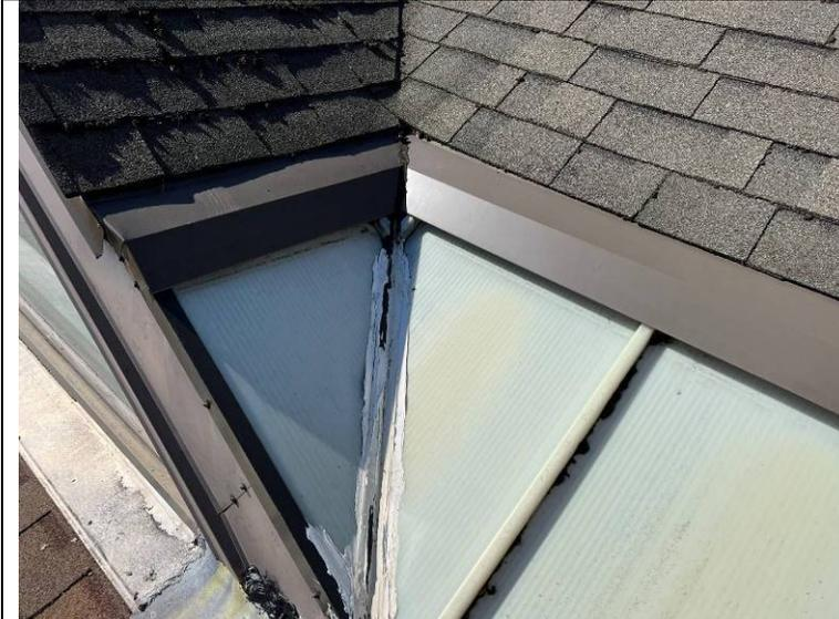
Photograph 53: Sealant at this location is older and was likely applied in response to previous water entry.
