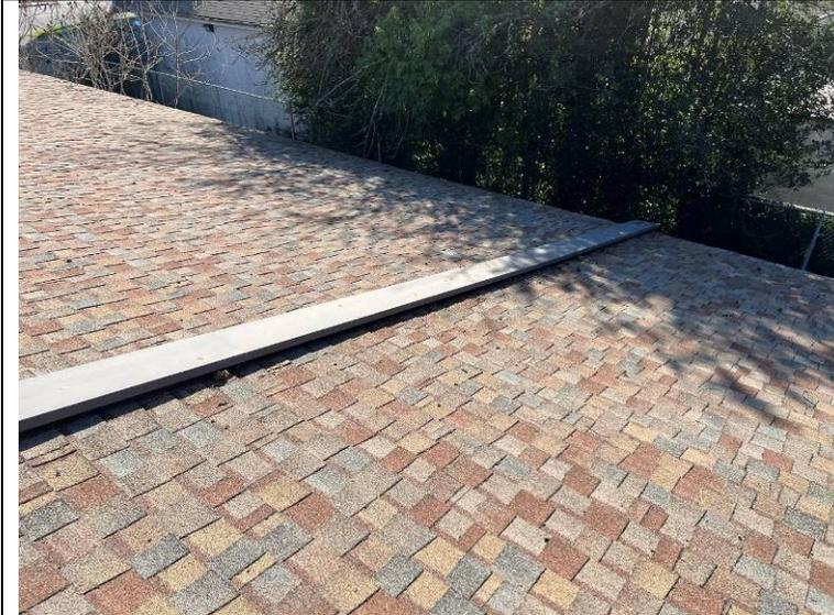
Photograph 38: Sheet metal cover over an area dividing wall.
