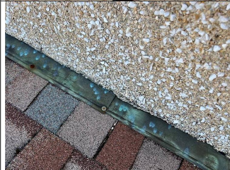
Photograph 33: Closer view of the headwall flashing.
