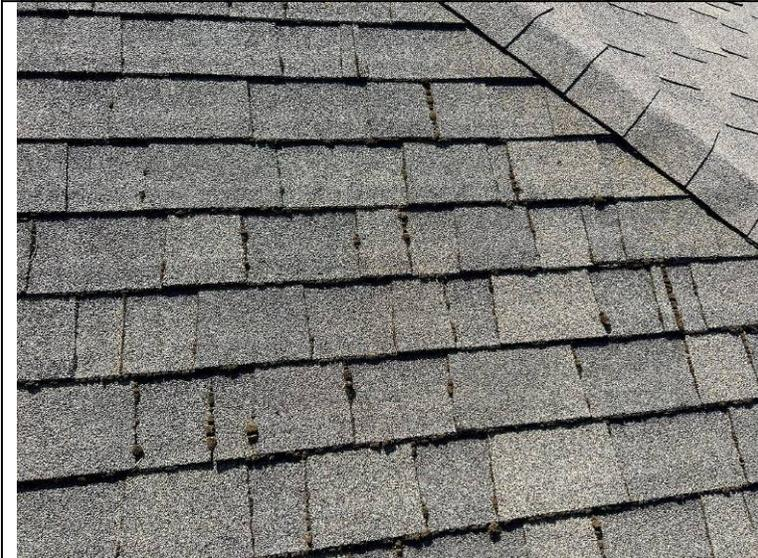
Photograph 90: Alternate view of the moss growth at the upper roof.
