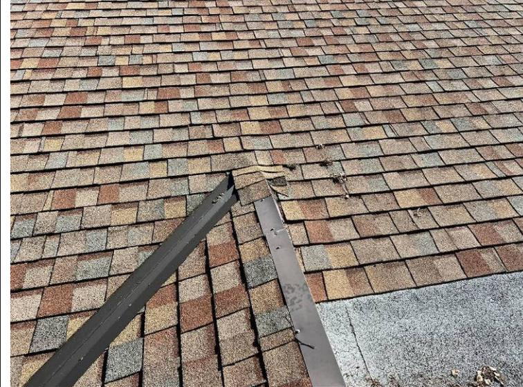
Photograph 83: Closer view of the steep slope to low slope transition.
