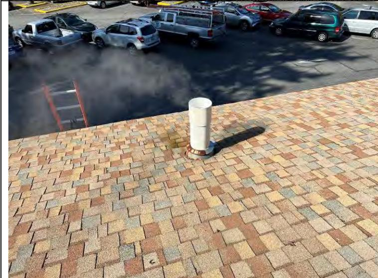
Photograph 65: Boiler vent penetration.
