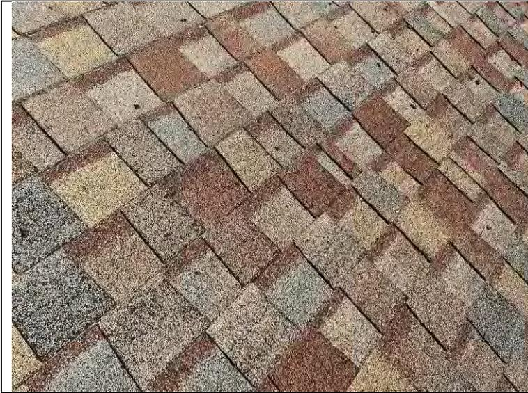
Photograph 61: At the south sloping roofs, the mineral granules are eroding from the surface of the shingles.
