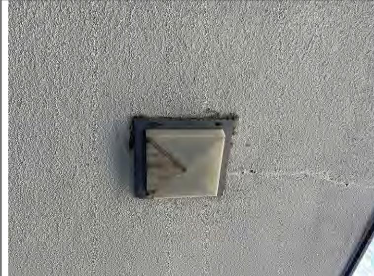
Photograph 5: Water staining at a light fixture in the soffit under the area where test openings were made.
