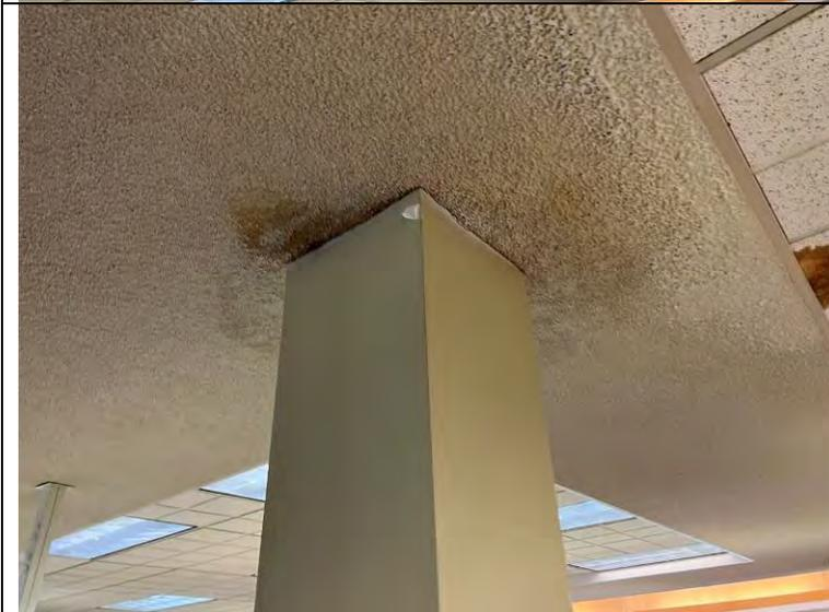
Photograph 81: Closer view of the stained ceiling in the general area shown in Photograph 79.
