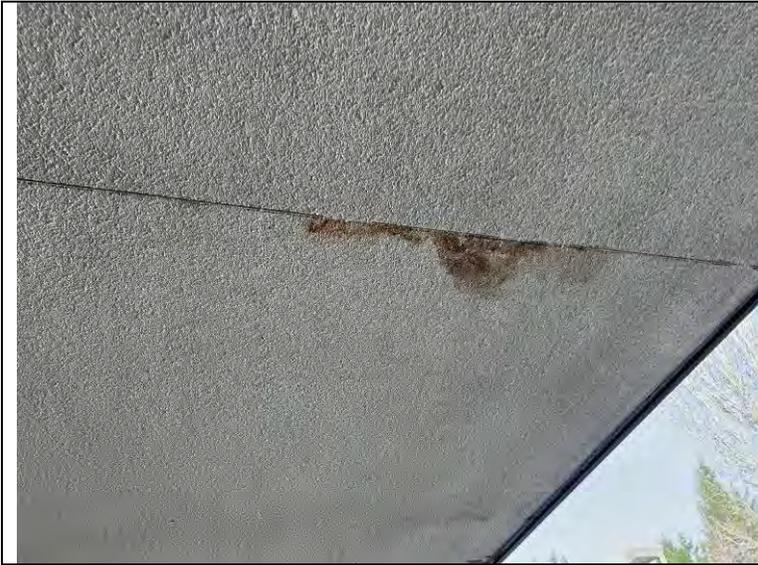
Photograph 7: Water staining at the soffit under the area where test openings were made.
