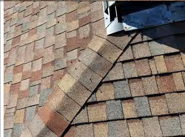
Photograph 47: Closer view of the backed-out nails.
