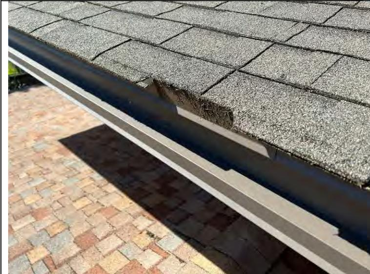
Photograph 104: Damaged shingle at the eave edge.
