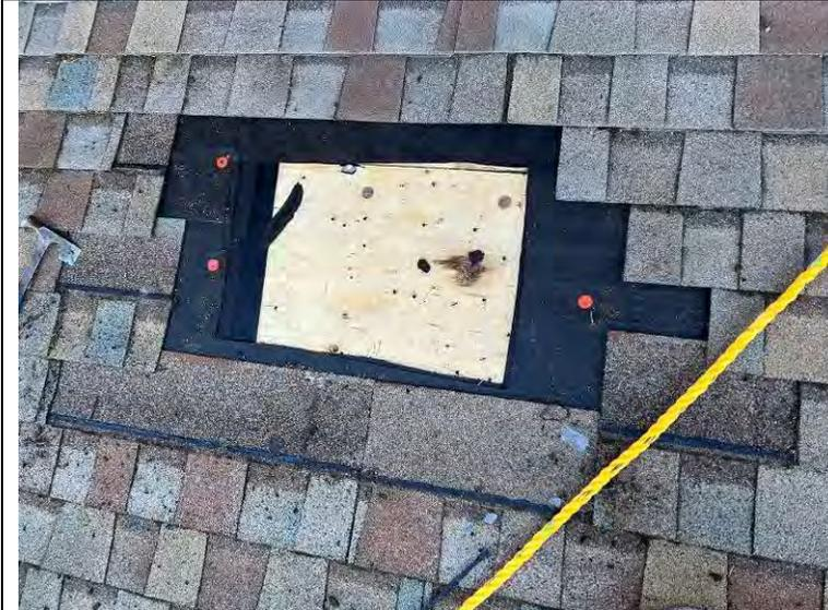
Photograph 8: Test opening #1 was situated under the overhang from the upper roof. The plywood at this location appears light in color and solid.
