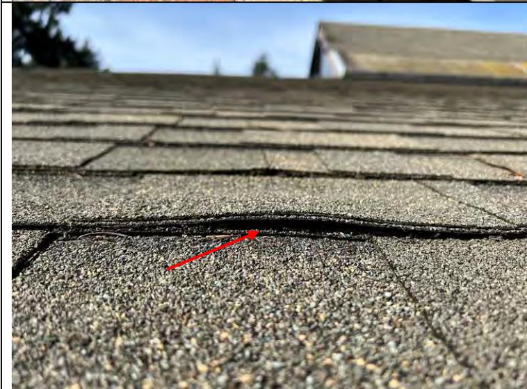
Photograph 105: Arrow indicates an apparent nail backing out and lifting the overlying shingle.
