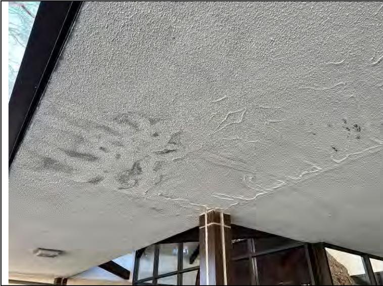
Photograph 4: Water staining at the soffit under the area where test openings were made.
