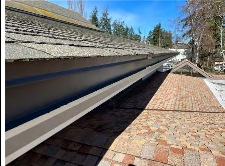
Photograph 101: Eave edge without a gutter.
