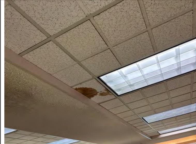
Photograph 80: Closer view of stained ceiling tiles shown in Photograph 79.
