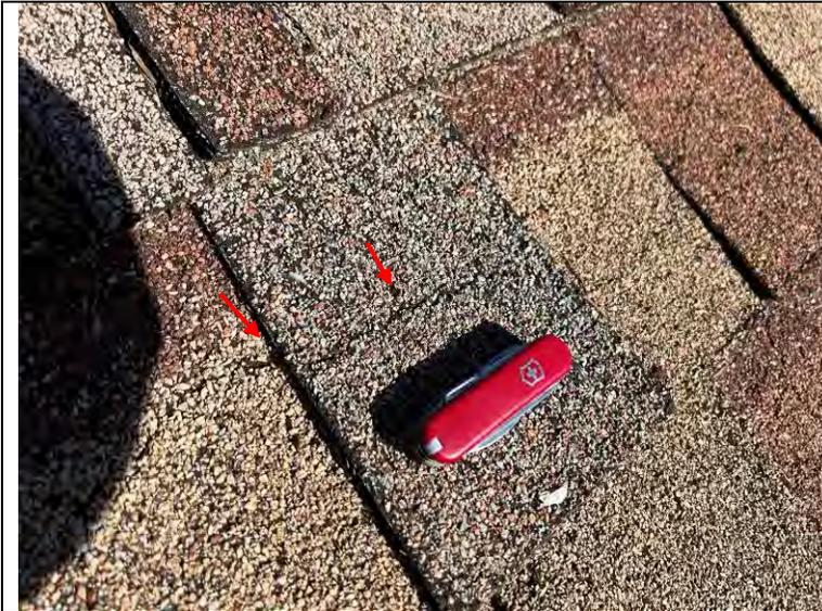
Photograph 64: Cracked shingles at the south sloping roof. (Arrows)
