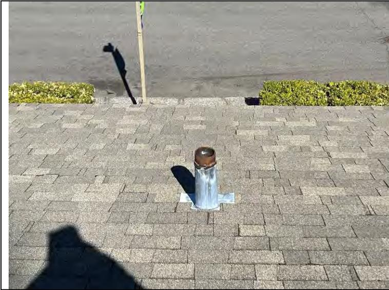
Photograph 97: Pipe penetration flashed with a lead flashing.
