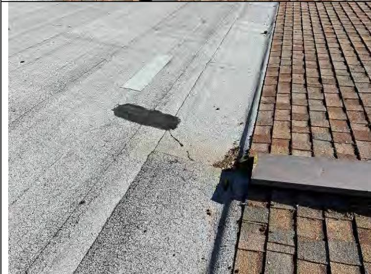
Photograph 78: Closer view of the roof cement patch circled in Photograph 77.
