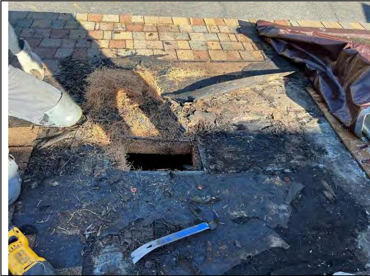
Photograph 13: Portion of the cementitious wood fiber substrate was removed to provide visual access to the structure below.
